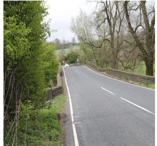
Existing carriageway looking East across the bridge
