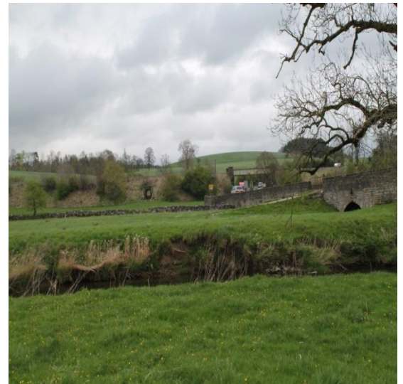
North side of causeway looking East towards the position where the new causeway will re-enter the existing carriageway.
