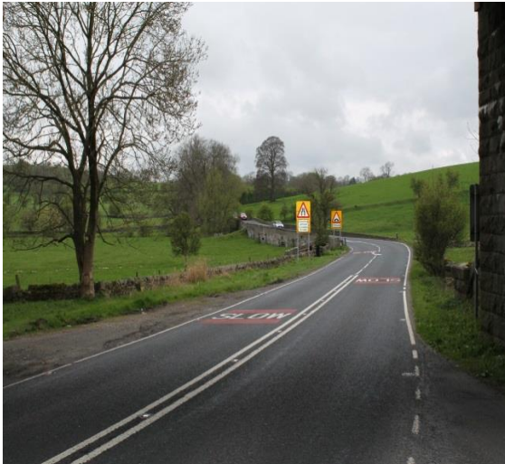
Existing carriageway looking West across the bridge
